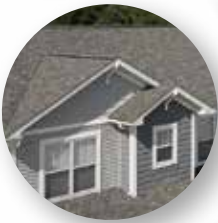
Roofing and Ventilation
